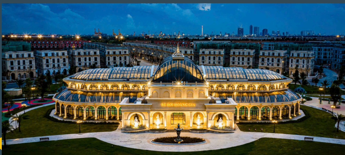
Vinhomes Vu Yen Project - Royal Island City (2025)
