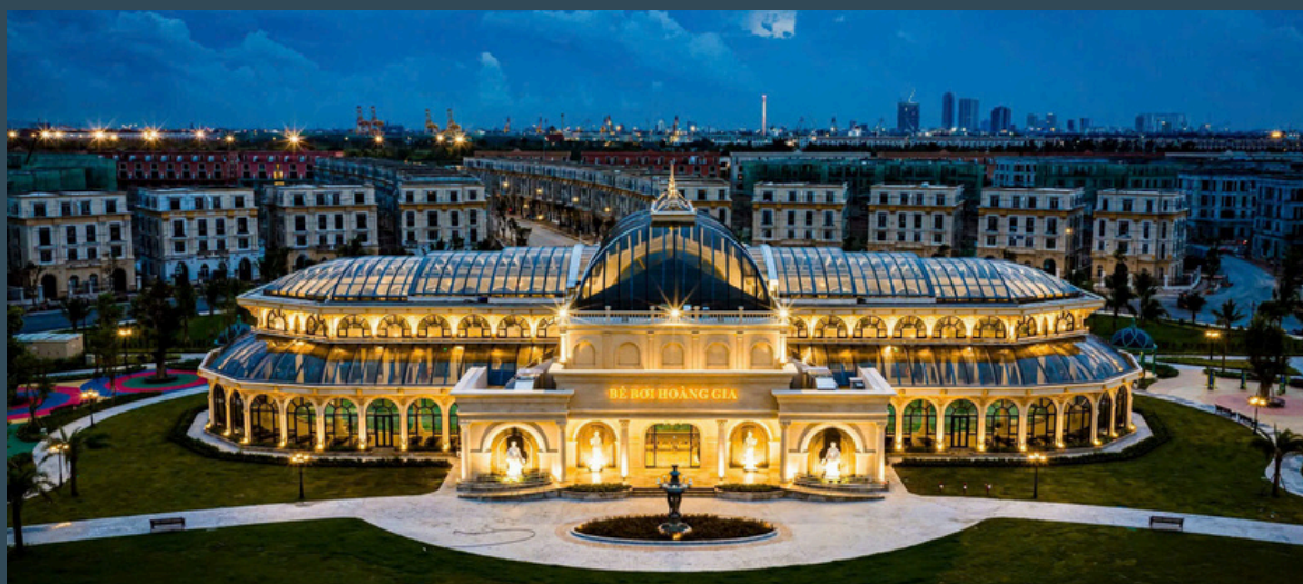
Vinhomes Vu Yen Project - Royal Island City (2025)
